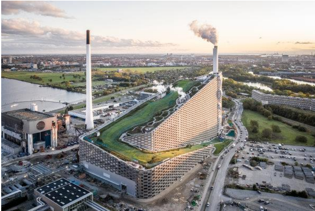
The Amager Bakke power plant in Copenhagen is topped with an artificial ski run. Its synthetic bristles aim to simulate a freshly groomed slope.
